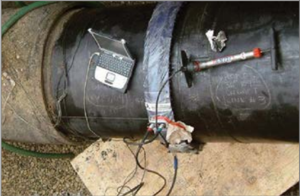
Inspection and Verification
