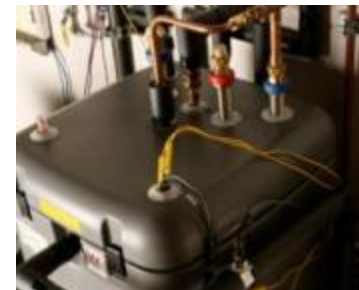
Equinox Solar-Assisted Heating System*
