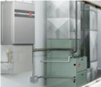
Water/Space Heater Combo System (90% + efficiency)
